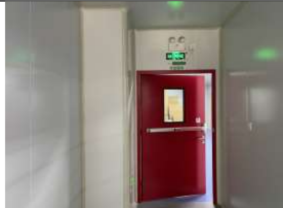
Corrected-Door with exit sign and emergency light
