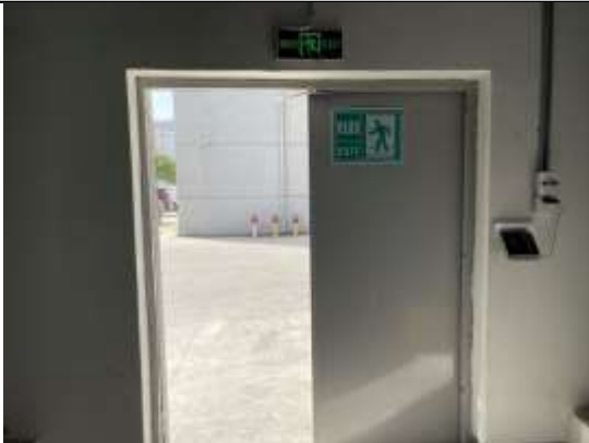
Corrected-Door open with single motion
